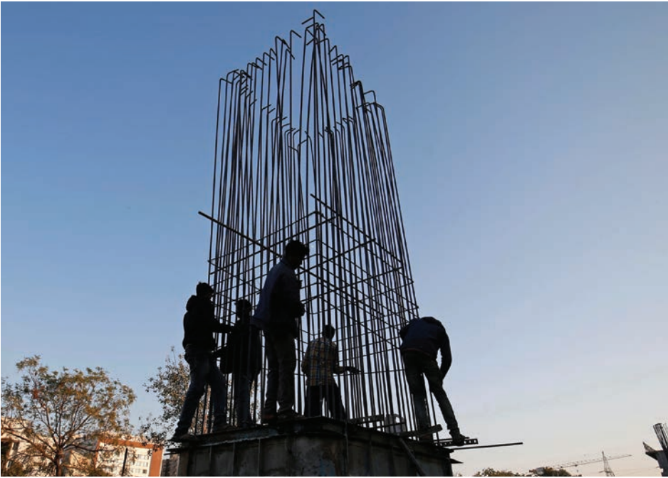
If you build it: highway construction in Ahmedabad, India, January 2021
